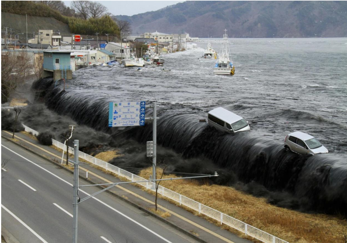
Tsunami overtopping seawall defence in Miyako, Japan, 11 March 2011 (photo from Miyako City Office via Reuters)
